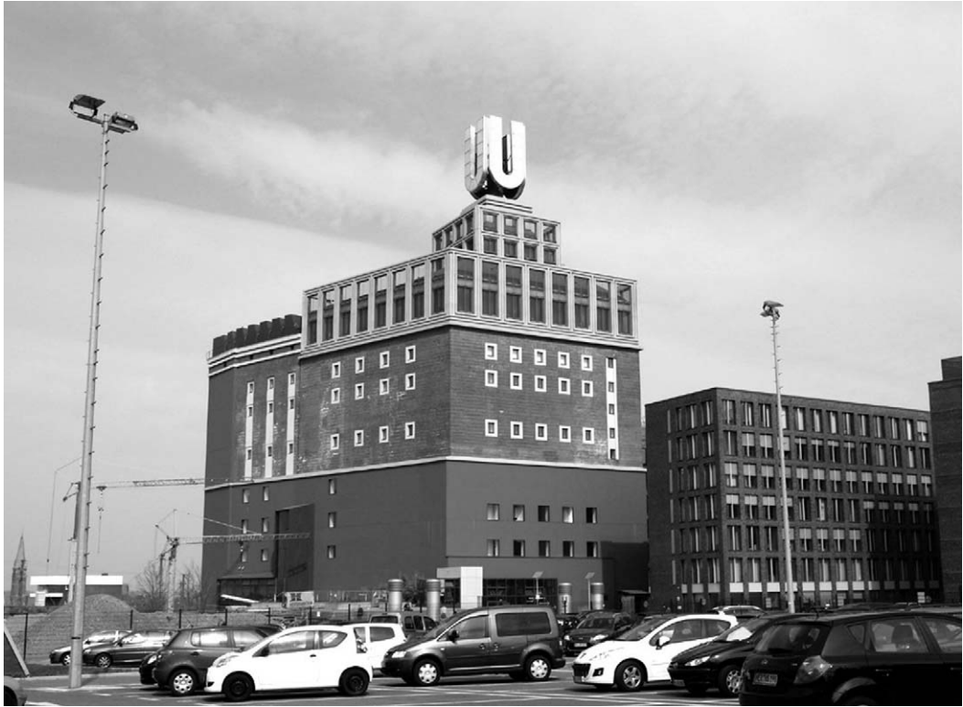
Figure 9: U-Tower after reconstruction and reuse as a center for arts and creativity. (Photo by the author)
