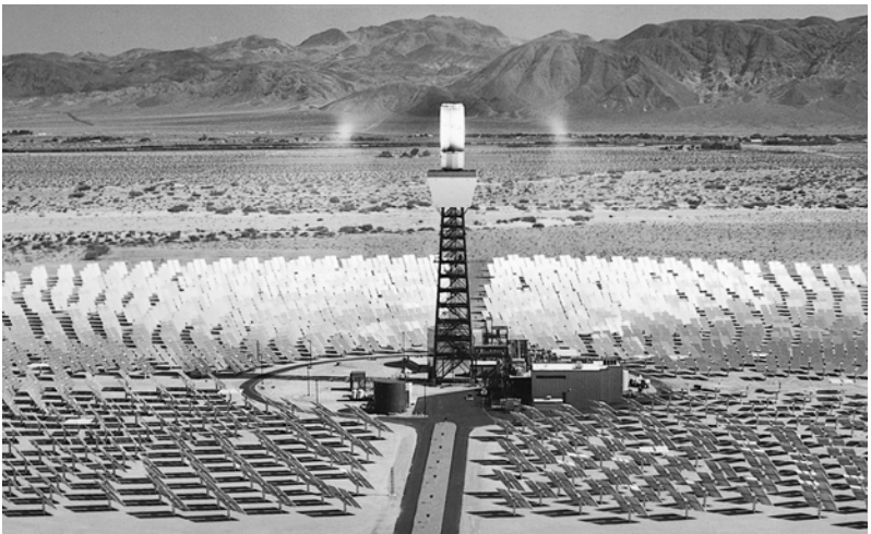
Figure 3-4. Solar One Power Plant located near Barstow, California. 5 In explaining the operation of this plant in a presentation, a logical strategy would be to follow the flow of energy through the system: Sunlight strikes the mirrors and reflects onto the receiver mounted on top of the tower. This radiant energy is converted to heat in a transfer fluid that flows to a turbine to produce electrical energy.
