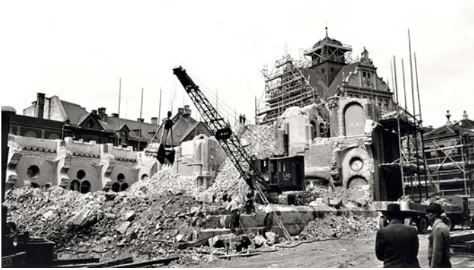
(Fig. 2) Demolition of the main synagogue, June 1938. Source: Stadtarchiv München
