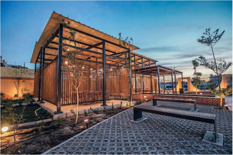
Figure 2. Pavilion rope partitions and surrounding permeable paving/pervious surfaces. Source: © Takween Integrated Community Development 2021.
