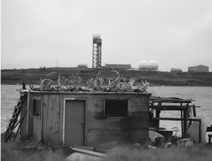
DEW Line radar station, Tuktoyaktuk, Northwest Territories, Canada. The Distant Early Warning (DEW) Line was a system of radar stations constructed along the northern coasts of Alaska and Canada in the 1950s. Additional stations were built in the Aleutian Islands, Greenland, Iceland, and the Faroe Islands. It was designed to detect Soviet bombers and missiles approaching North America via the Arctic. By the 1980s, advances in military technology soon rendered the system obsolete and many stations were decommissioned and abandoned. Some stations were upgraded as part of the new joint US-Canada North Warning System in 1985. Photo: Mark Nuttall.
