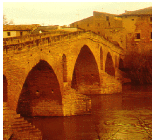
The Romanesque bridge in Gares (Navarre, 11th century)
