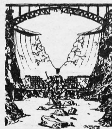
GLEN CANYON DAM
