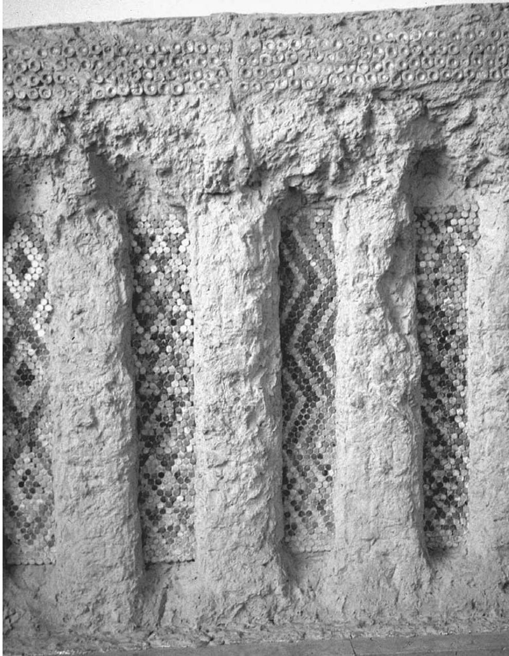
Part of the clay brick wall of the ancient Sumerian city of Uruk, displayed in the Pergamon Museum, Berlin, is decorated with colored terra-cotta cones. It may serve as a metaphor for the separation of the city from its rural and natural environs. (Photo courtesy of J. Donald Hughes)
