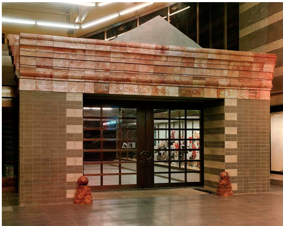
Figure 6 Ján Bahna, portal, Ružinov Shopping Mall, Bratislava, 1978–84 (Archive of Ján Bahna).
