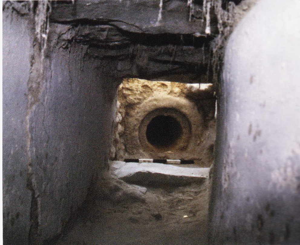
Terminus of stone pipeline and beginning of the masonry channel
