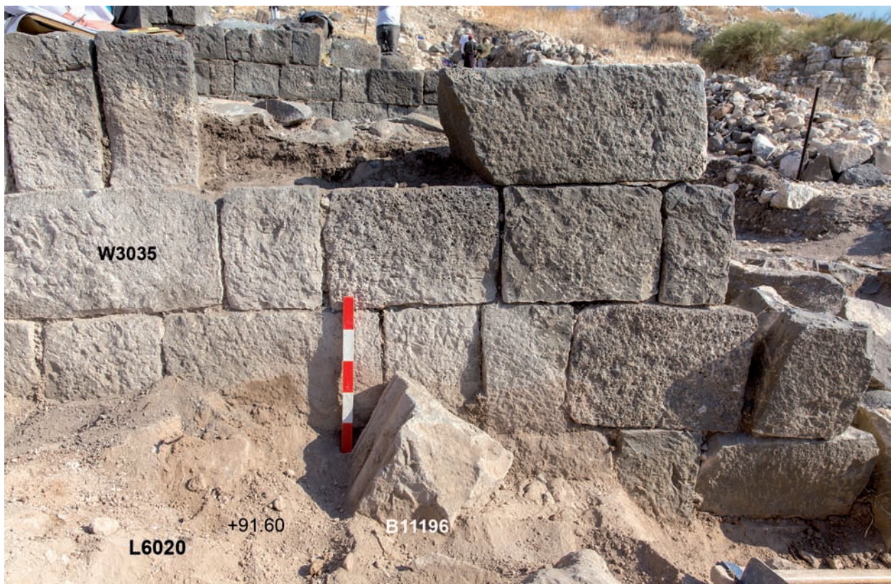
Fig. 18. The propylaeum. The western wall of the western tower. Note one of the profile stones in its outer debris and the wall's collapse in its southern part. View towards east
