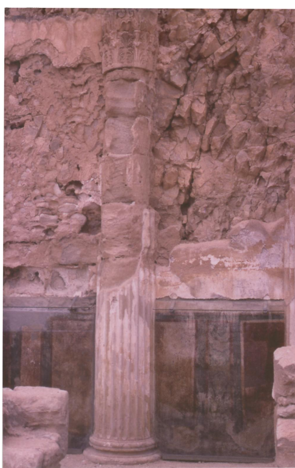
All of Herod's palaces were lavishly decorated. This photo shows the painted plaster from the lowest terrace at the Northern Palace. The artists painted the plaster to appear to be marble. Photo courtesy of D. Hopkins.
