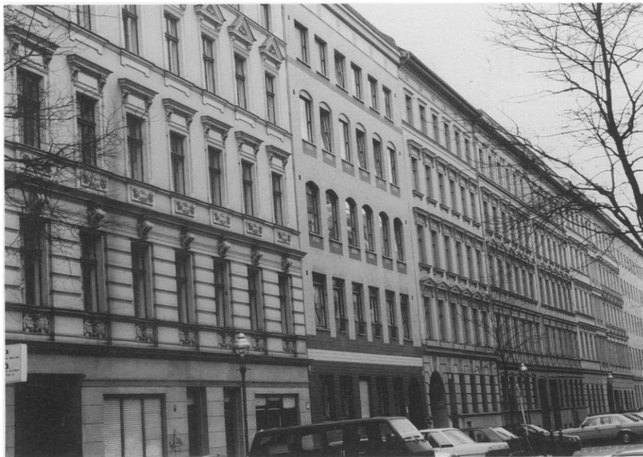
6. Liebenwaldstrasse 57-50 (1994) "New" Mietskaserne No. 56 second from left.
