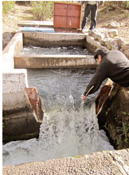
The water flow rate in the canal valves is measured through standardized hydraulic outlets.
