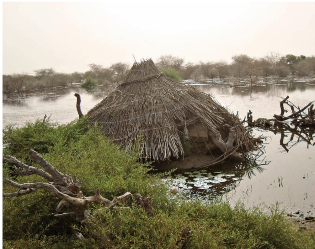
Granaries close to Mare d'Yomboli collapsed due to severe flooding in 2010.
