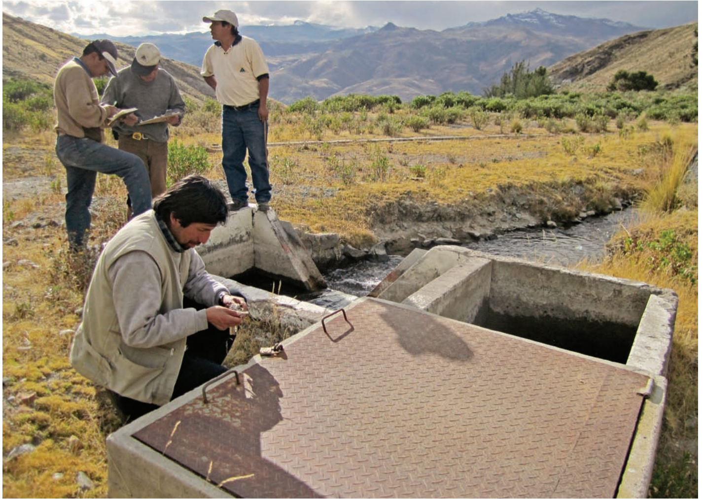
The engineer working for the Water Users' Organization in Colca Valley is the keeper of the valve keys.
