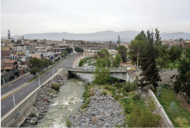
Regulated flow of water streaming through the Chili River.
