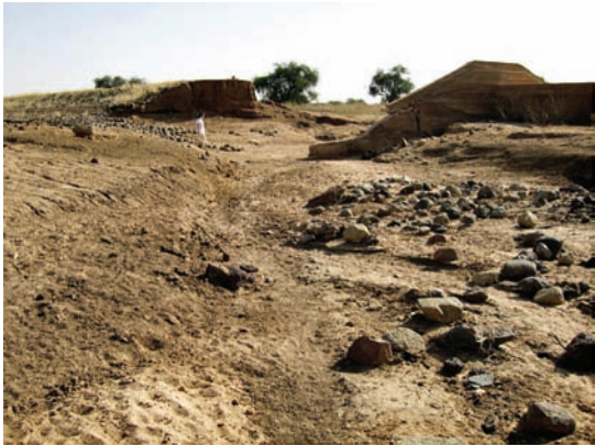
The dam made for the rice irrigation scheme – one year after it was destroyed by a tropical rainstorm.
