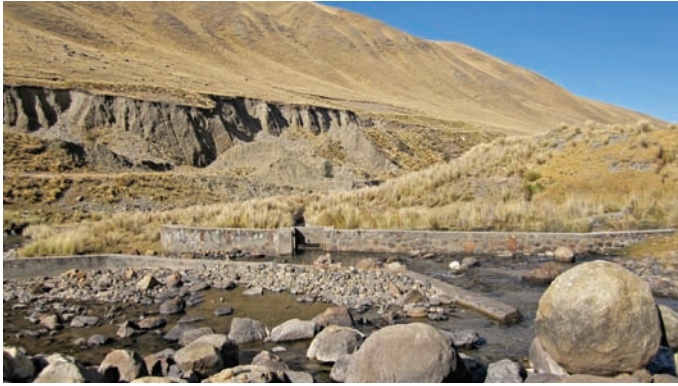
The intake constructed in 1996 bears the name of the then president Fujimori.
