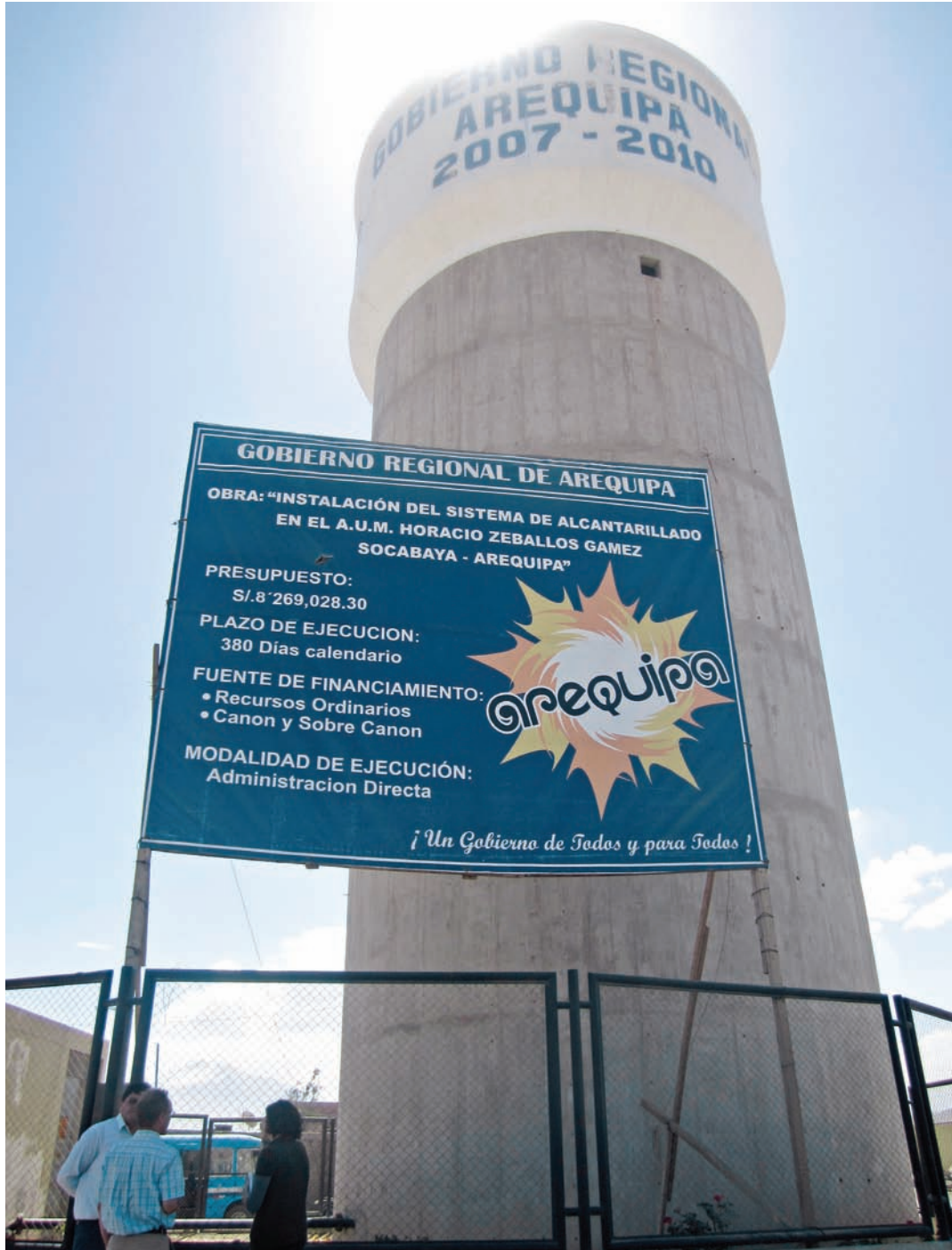
Water tower in Machabaya. Sign with logo of the regional government of Arequipa.
