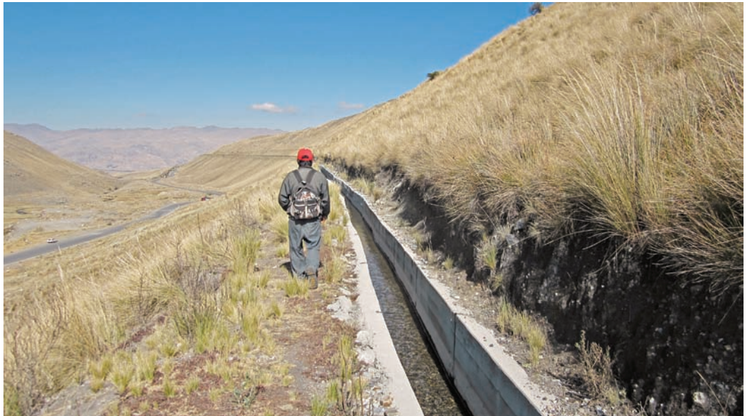
Don Seferino balancing on the concrete that lines the first part.
