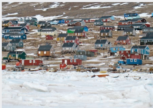
Houses in Qaanaaq, built on wooden poles and permafrost. This technology is gradually melting down, and houses begin to slant.
