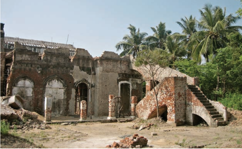
The Danish Governor's bungalow before restoration.
