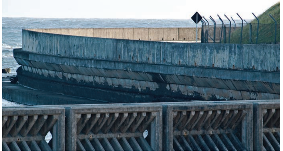
Sea wall and wave breaker outside the international airport.
