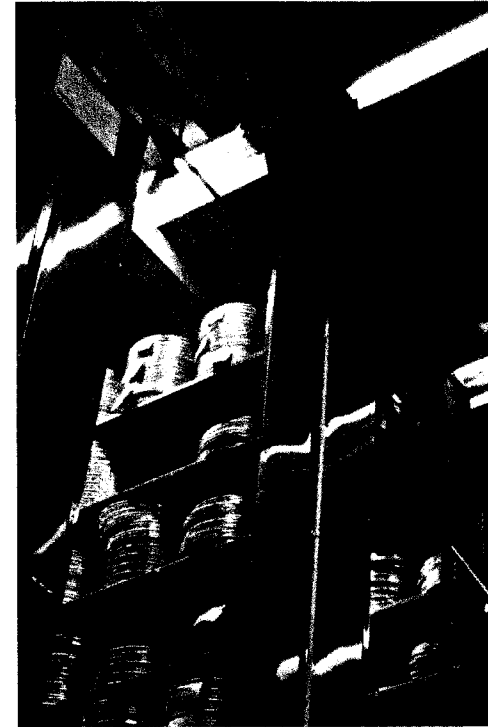
Figure 2.1 An atmospherically controlled vault at the British Film Institute's conservation centre near London. Air that has been treated to achieve a consistent temperature and humidity is pumped into the space through the one-way membrane mounted on the ceiling above the fluorescent lights. The BFI's Harold Brown discovered that cool and dry storage inhibits the decomposition of nitrate and acetate film base, and dye-coupler colour film emulsions, thereby enabling their long-term storage in a passive conservation approach.
