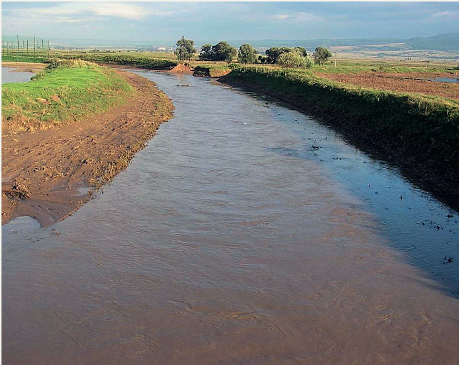
Fig. 15. Straightening of the Lesnovksa River in Ravno Pole
