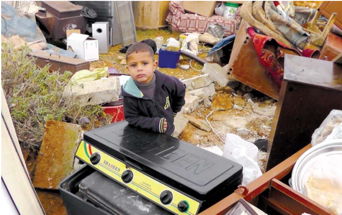
Demolition of Ka'abneh home, village of Beit Hanina al-Balad, north of Jerusalem. Photo: Iyad Hadad, B'Tselem, 24 November 2011.
