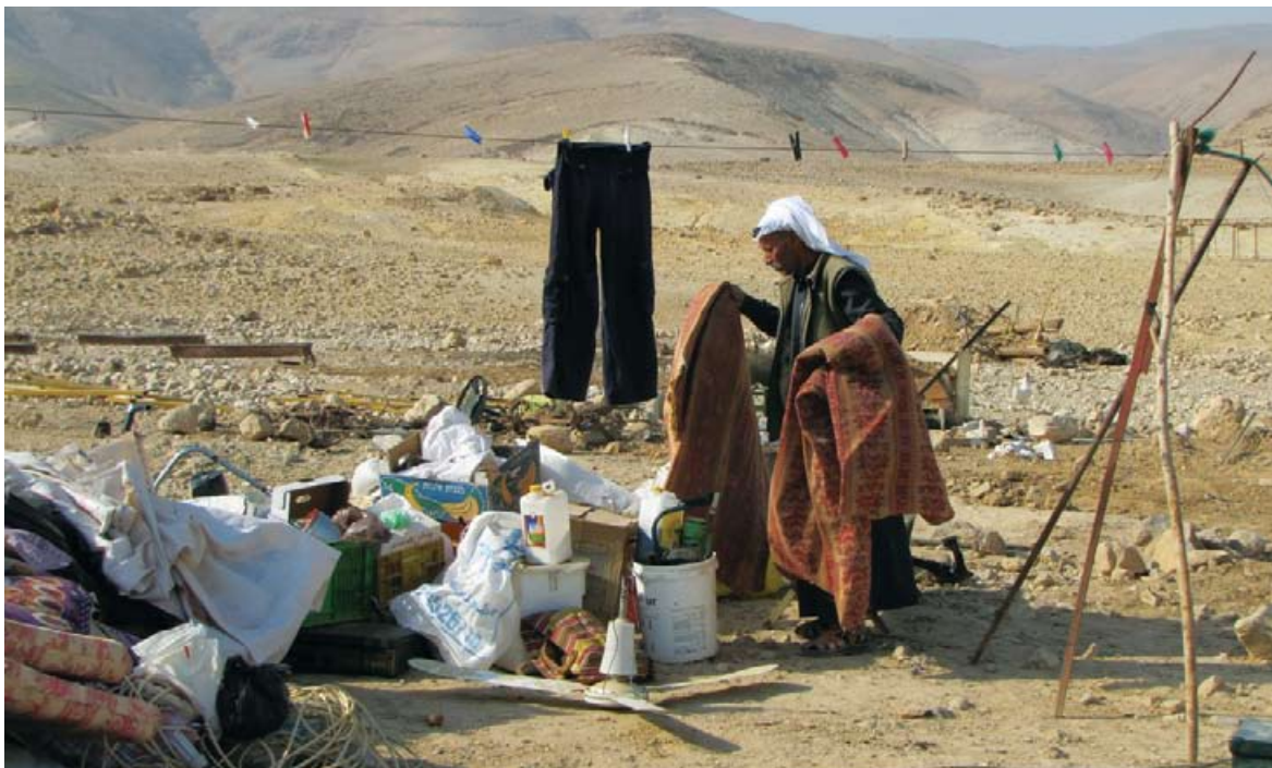
Demolition of homes, Fasayil, the Jordan Valley. Photo: 'Atef Abu a-Rub, B'Tselem, 20 December 2011.
