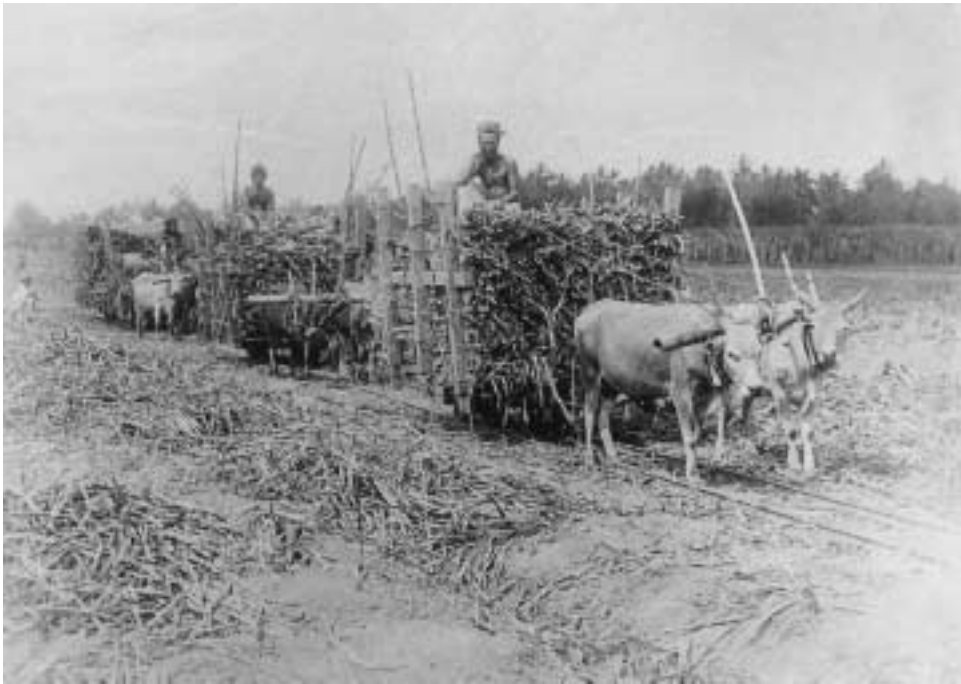
Figure 2 Western technologies were often mixed with local technologies to create new hybrid systems. In the early 20th century, the transport of sugar cane in the Dutch Indies was done combining domestic means with a rail track.
