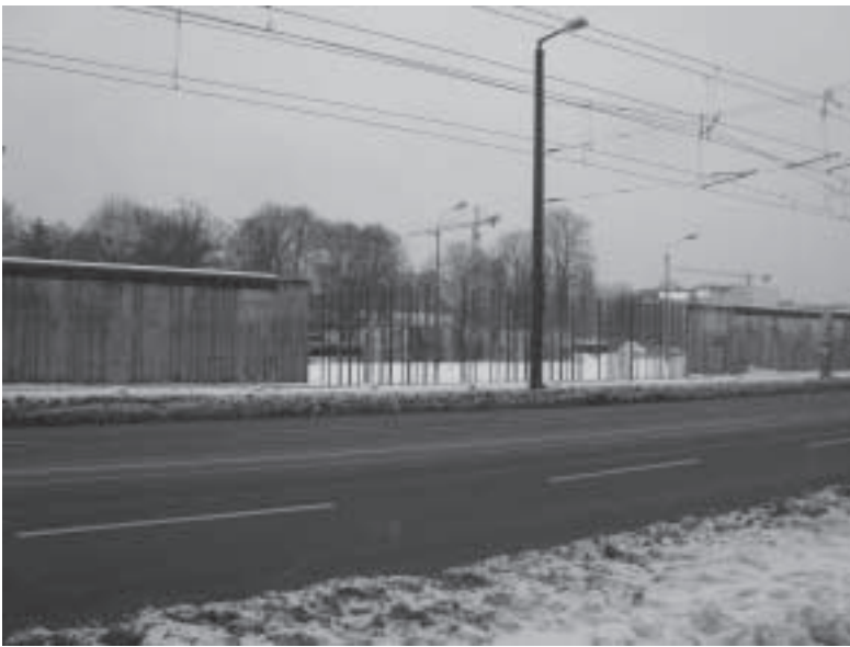
Figure 3: The Hole in the Wall Filled in with Corten Steel Posts
