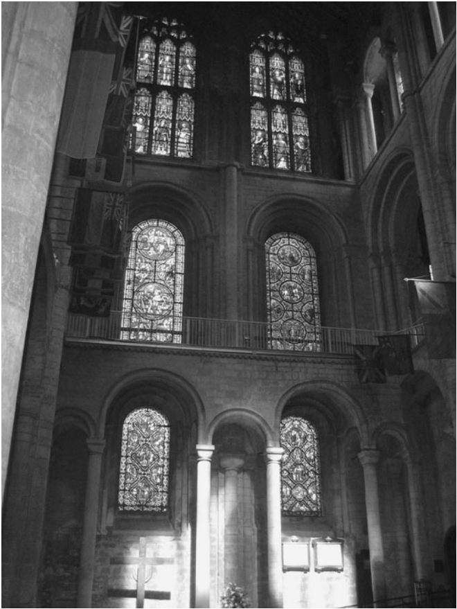
9. Ely Cathedral (then Abbey): it is just possible to detect the break in building during the vacancy between 1093 and 1100, when the abbey was in the king's hands. The break runs from the north-east corner of the north transept to the easternmost bay of the south aisle of the nave
