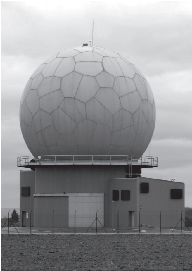
Newly built NATO air-defense radar base near Nepolisy, some 85 kilometers east of Prague, Czech Republic, photographed on January 20, 2007. Under President George W. Bush, the United States proposed installing components of its own missile defense system in the Czech Republic, a suggestion denounced by Moscow. (AP Photo/CTK, Alexandra Mlejnkova)
