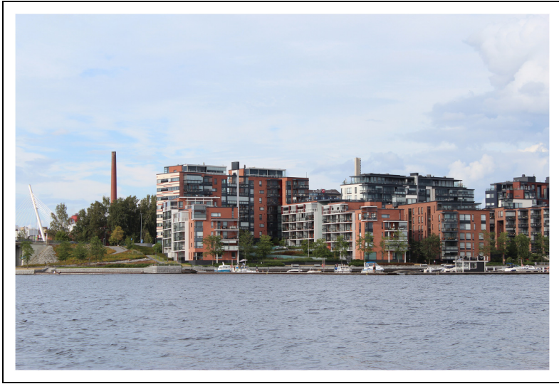
Figure 4. Ratina is remade on a brownfield site. Photo Antti Wallin.
